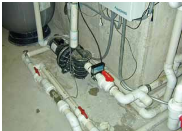
TOPS installed the new conditioning system in an effort to decrease the use of chemicals to control water quality.
